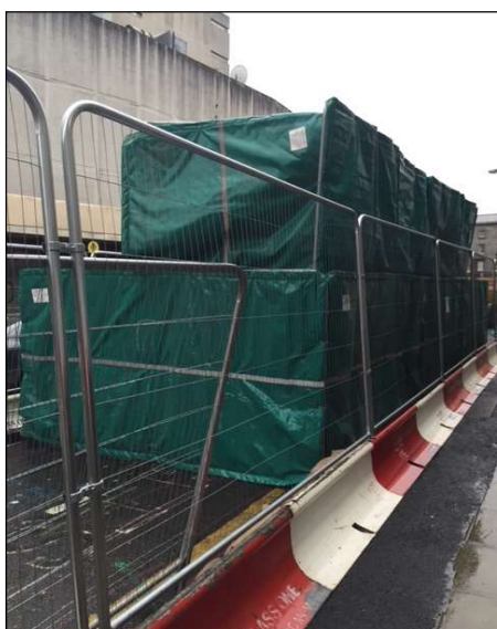
Double height acoustic blanket enclosure
