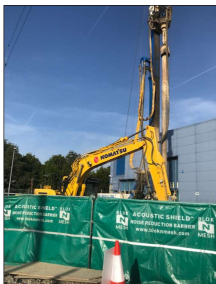
Acoustic blankets screening excavations
