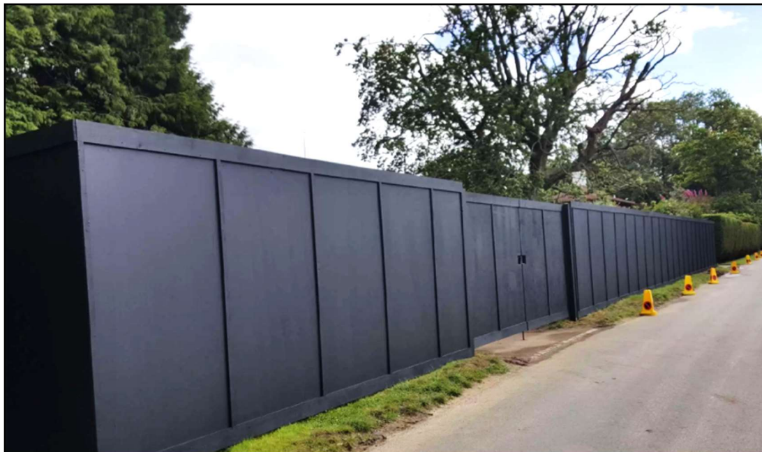
Photo 2 – Typical Site Hoarding Arrangement
